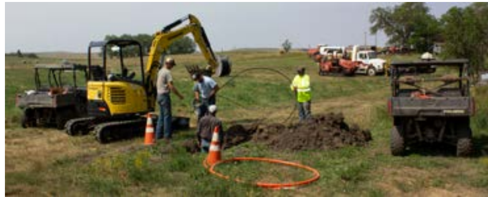
Construction on-going to deliver high-speed Internet to the Town of McIntosh. 788-2822
